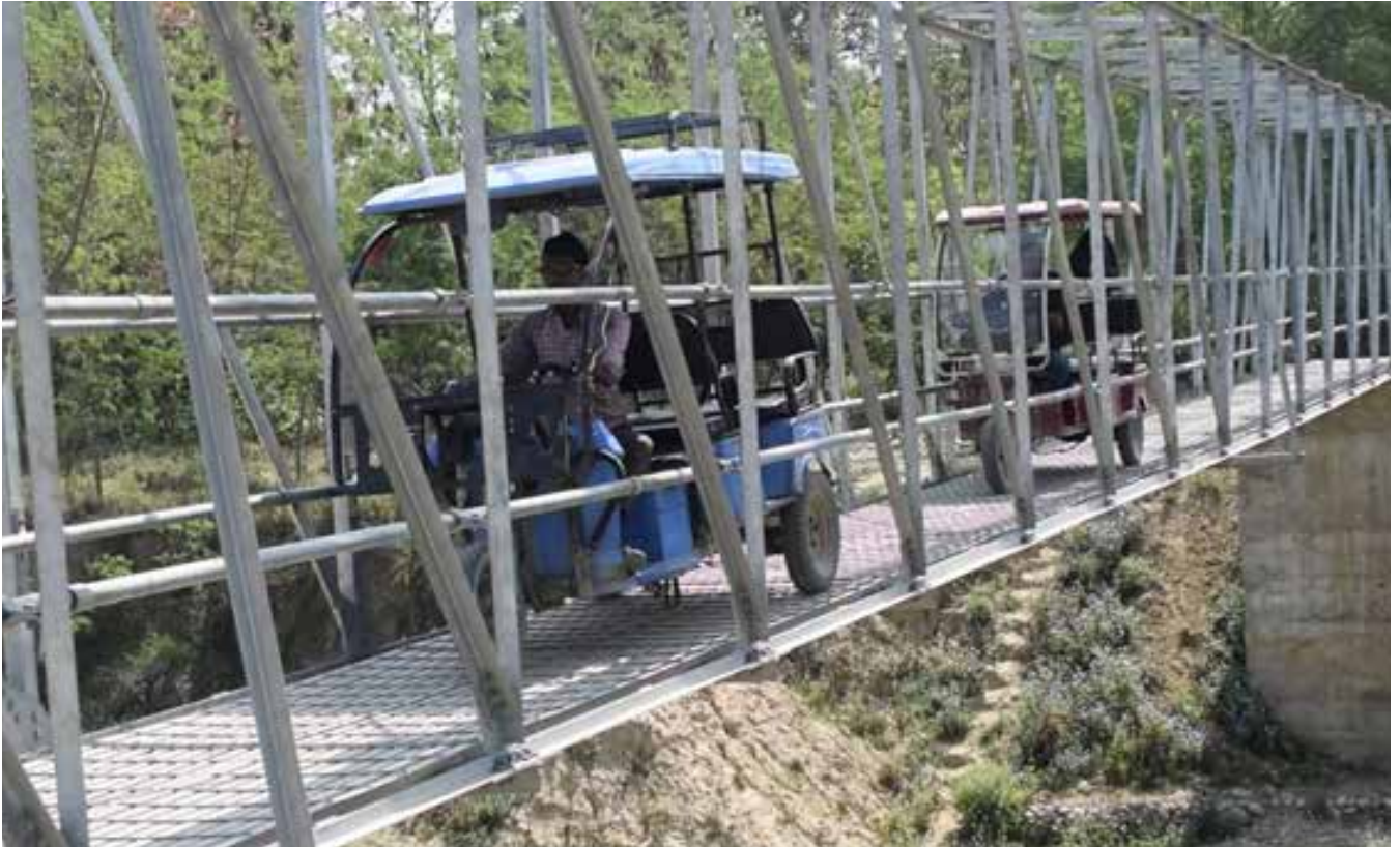
Capacity to accommodate E-rickshaws is an added value of Teshanpur bridge, Bardiya
